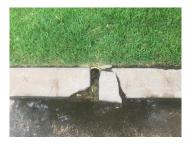
This is a section of curb around where the property owner cut through the curb to make an exit for a French drain. The Facilities Committee has long taken the position that we do not accept responsibility for these, as they were all added after the house was built, thereby negatively impacting the structural integrity of the curb. While these areas should be repaired, we do not accept responsibility for these repairs.
