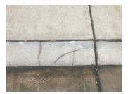
In this case I kicked the curb and nothing moved; so, I concluded the rebar is holding things together reasonably well and will probably defer repairs.
